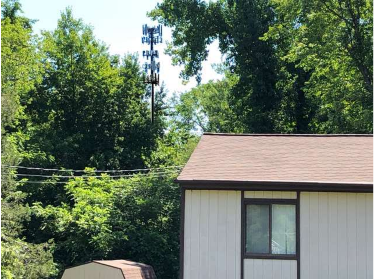
110 Caroline Drive East - Tarpon Tower Balloon Test - View from front lawn with balloon at 150 feet high. Includes view with cell tower being proposed at the 150 ft balloon test height...(it will be built to 170ft if approved)
