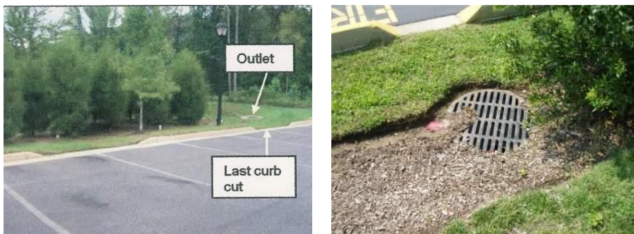
Figure 9.11. Examples of Short-Circuiting at Bioretention Facilities
