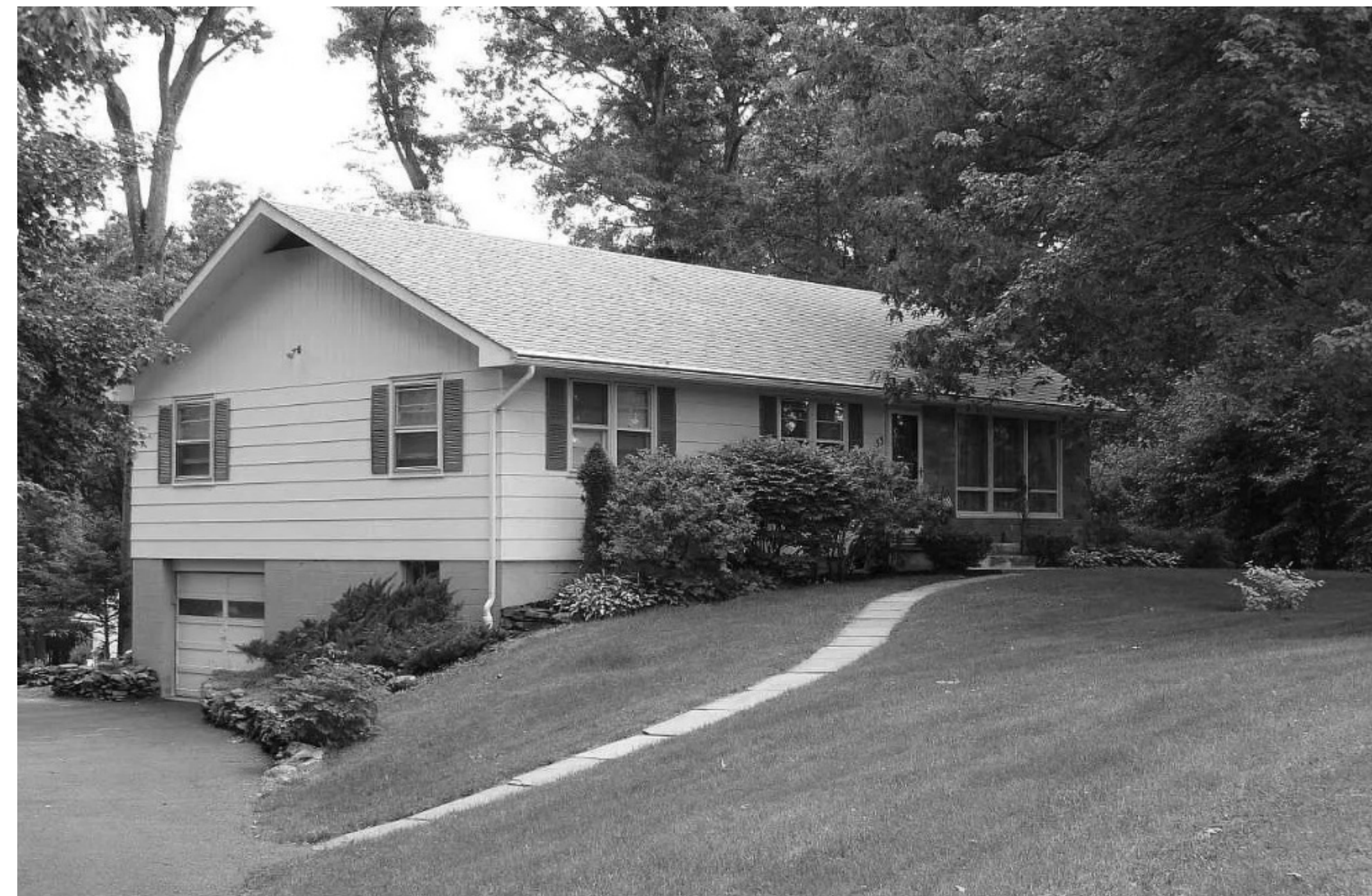
4 EXISTING PHOTO LEFT 3EX1.0 1/4" = 1'-0"
