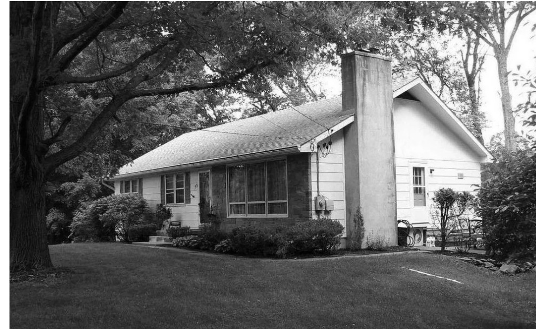
3 EXISTING PHOTO RIGHT 3EX1.0 1/4" = 1'-0"
