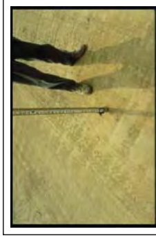
Fig. 3. Construction site with significant compaction of the deep basal till subsoil extends 24 inches below this exposed cut-and-fill work surface.
